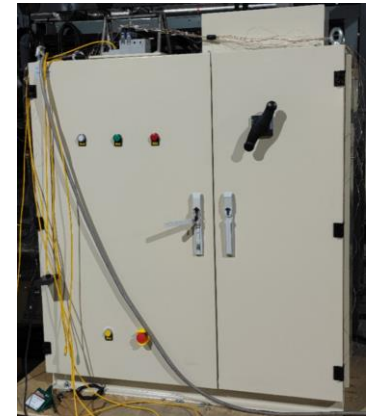
800kW Semi sealed/fully sealed 半密封/全密封
