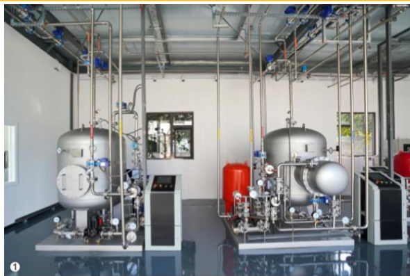
HEAT EXCHANGE EQUIPMENT & INTEGRATED HOT WATER SYSTEM 换热设备&集成热水系统
