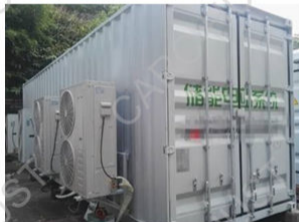
12.5kW分体式空调
